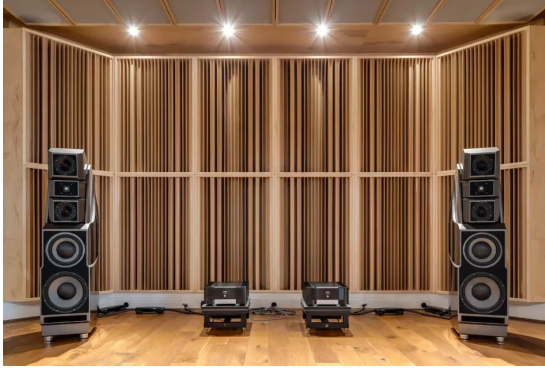
FIGURE 6.1. Quadratic residues are used in the design of echo-reducing wall panels for recording studios and concert halls. (Image: Dennis Foley, acousticfields.com)
